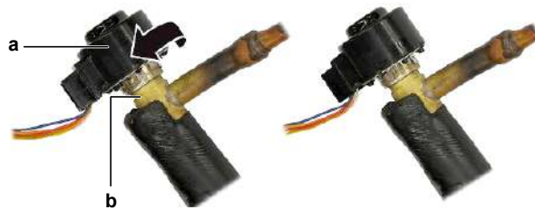
a Expansion valve coil b Pipe
